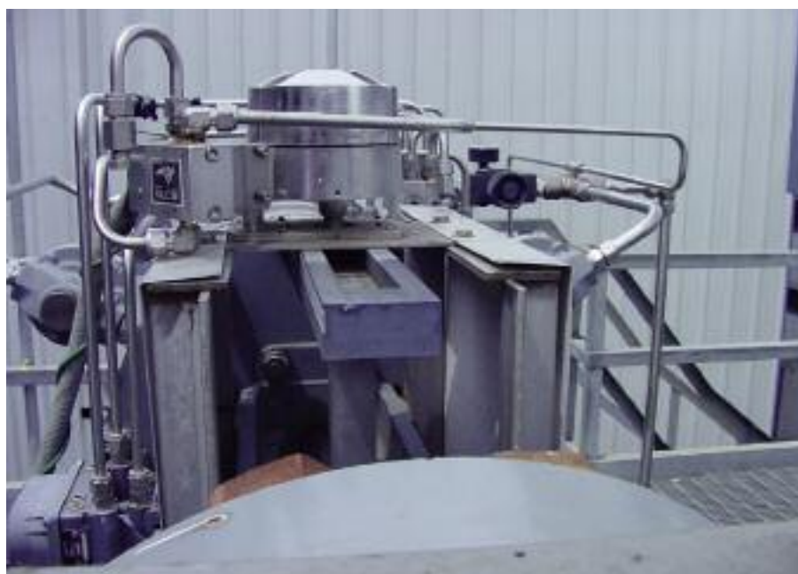
FIGURE 5—TYPICAL APPLICATION/DIGITAL CONTROL TRANSMITTER
